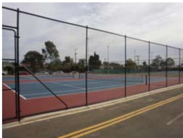
Courts at the Southern end
